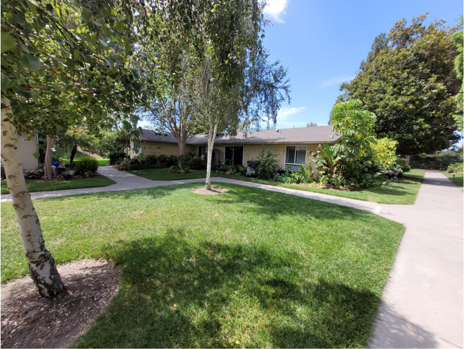
VIEW FROM WALKWAY FACING SOUTH TOWARDS REAR OF MANOR 196-A PIC #3
